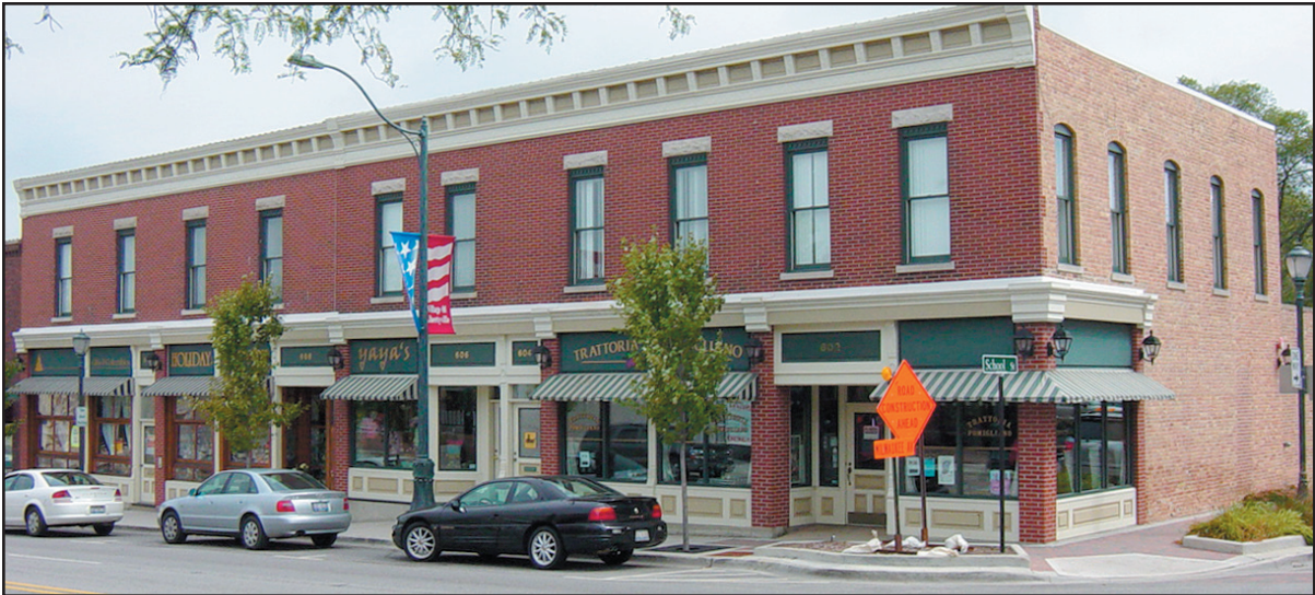
Example of distinct, recognized storefronts at base of mixed-use building.
