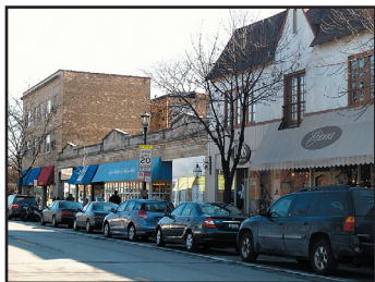
Retail and mixed-use buildings across from Independence Park at Central and Stewart.
