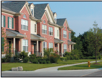
Rowhomes with landscaped front yards and attractive, articulated facades.
