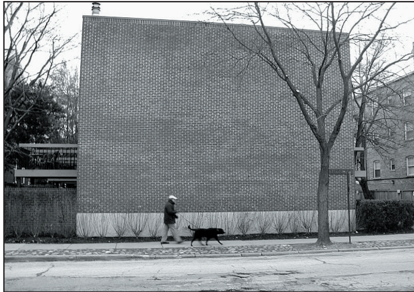
Some residential buildings near Ashland have blank walls that front the street.
