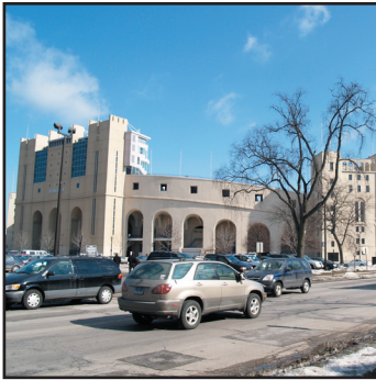
Northwestern University's Ryan Field, located at Central and Ashland.
