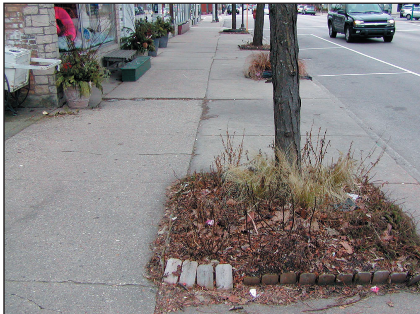
Poor tree pit conditions.
