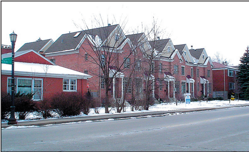
Recently constructed townhomes east of Bent Park on Central.
