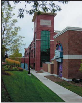
Example of structured parking with attractive facade located behind a restaurant.
