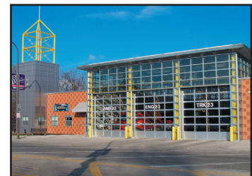
Fire station #3 at Central and Girard.
