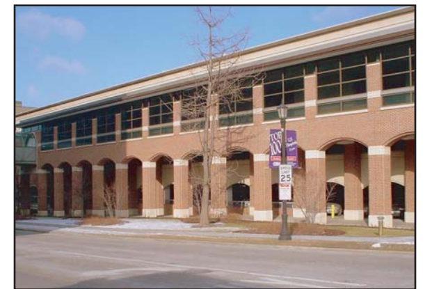
D Evanston Northwestern Hospital parking facility
