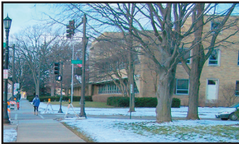
Office building at Central and Asbury.
